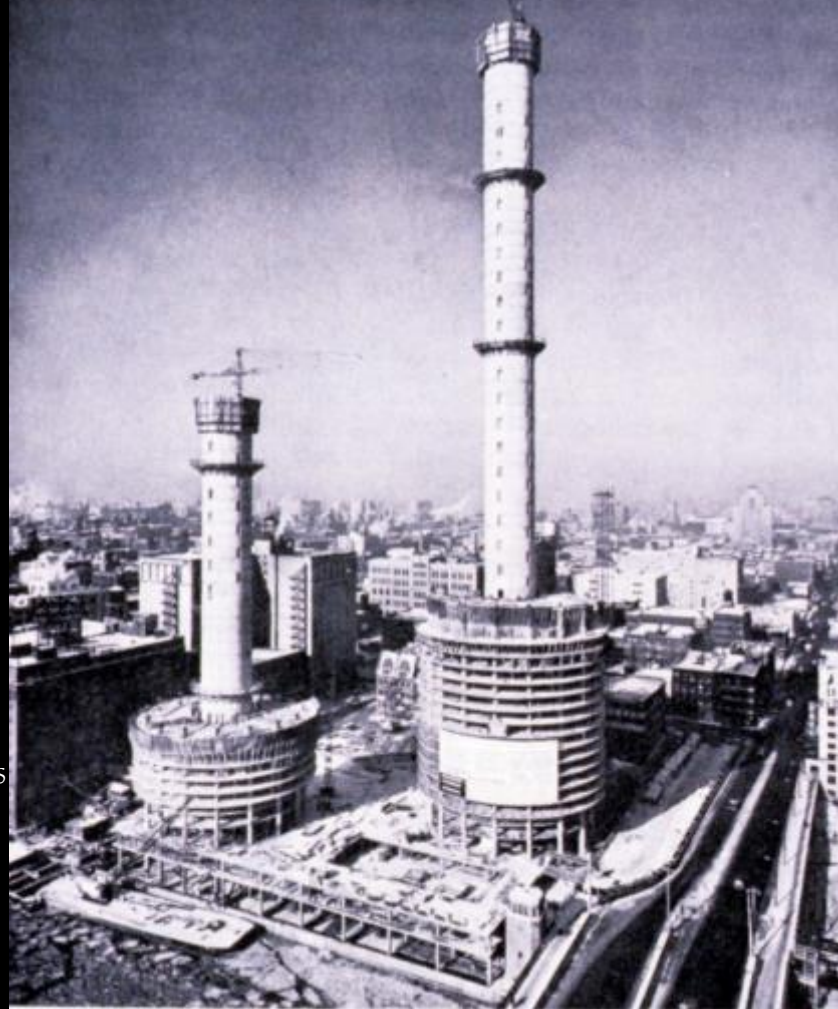
FIGURE 7.18 Marina Towers in Chicago during construction.
